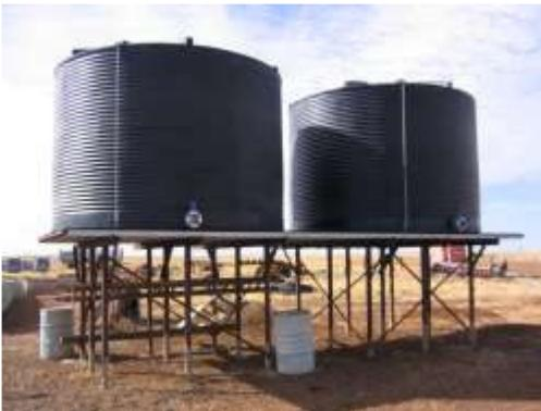
Poly molasses tanks are suitable for this system. If you only require a small amount of storage a 5800 gallon tank which holds approximately 36 ton of molasses is most suitable. Therefore, the stand needs to be built to accommodate this weight.
